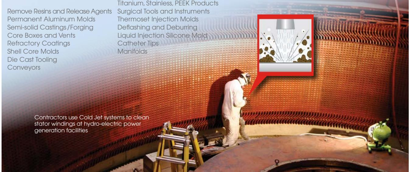
Contractors use Cold Jet systems to clean stator windings at hydro-electric power generation facilities
