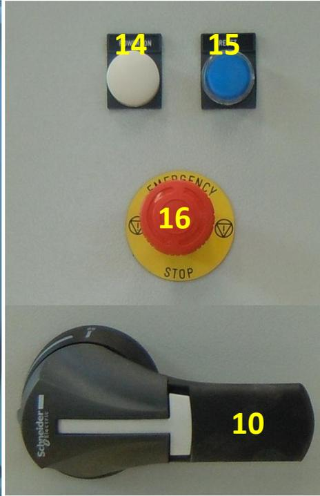
Figure 7 Control Panel Exterior
