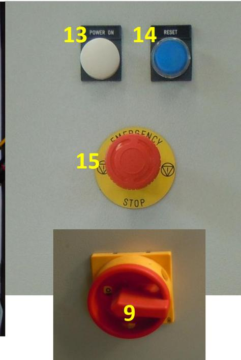
Figure 8 Control Panel Exterior
