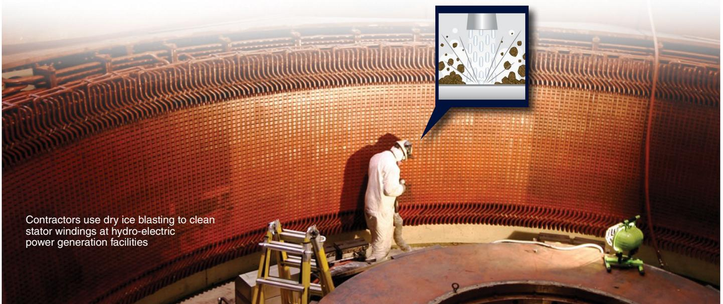
Contractors use dry ice blasting to clean stator windings at hydro-electric power generation facilities
